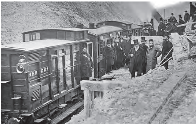
A landslide occurred at the Warren (Folkestone) in 1877, closing the line for three months and destroying over 100 yards of the Martello Tunnel. The official reopening is seen here. Alongside the train are Mr. Newborn (director), Hon. James Byng (director), Sir Edward Watkin (chairman), Mr. John Shaw (secretary), Mr. Charles Sheath (clerk to the chairman) and the guard is Mr. George Privet, who later became one of the SER's first two district superintendents.
